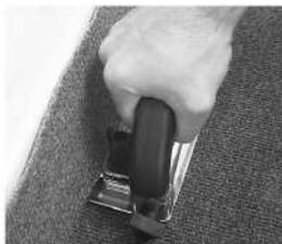
2. Keeping the base plate flat on the carpet and the guide bar against the wall, make the trimming cut.
